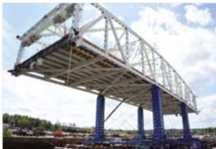
Incremental bridge lifting
