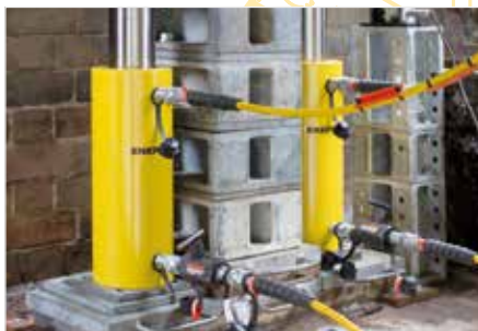
Bridge lifting and launching
