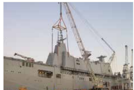
Synchronous hoisting and load positioning
