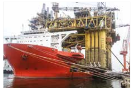
Synchronous superlift and launch
