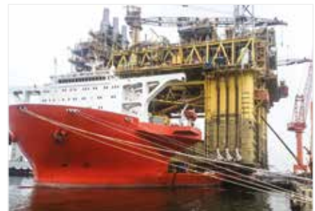
Synchronous superlift and launch
