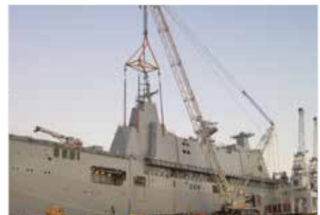
Synchronous hoisting and load positioning
