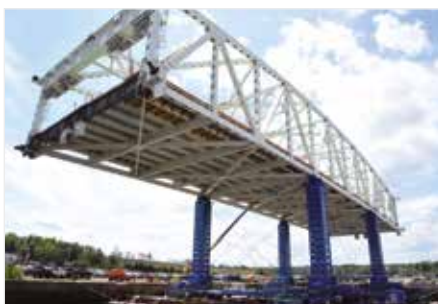
Incremental bridge lifting
