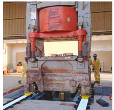
▲ Low-Height Skidding System Skidding used to remove an old press to make room for new equipment.
