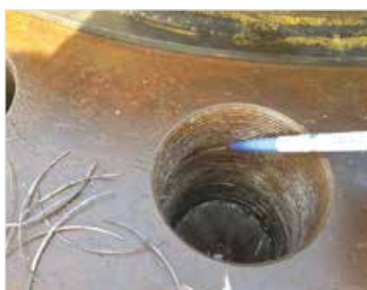
▲ A typical thread before refurbishment.
