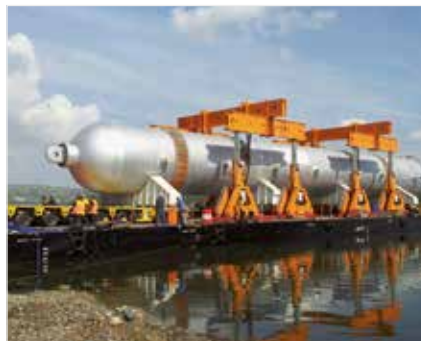
Using two SBL1100 gantries for offloading a 1300 tons hydrocracker
