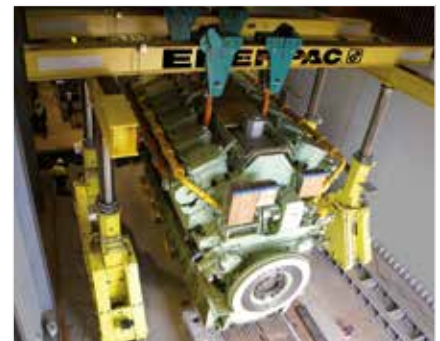
SBL1100 used for installing three 10.9 Megawatt diesel gas generators at the Owen Springs Power Station.
