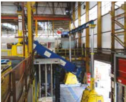
Transporting a 1200 tons hydraulic press to the second floor with a hydraulic gantry.
