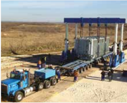
Transformer installation with a hydraulic gantry.
