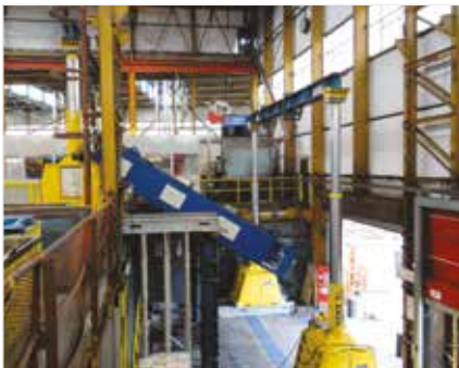
Transporting a 1200 ton hydraulic press to the second floor with a hydraulic gantry.
