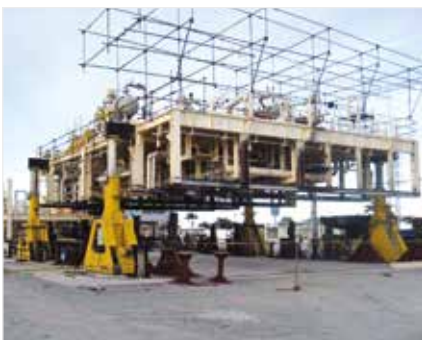
SBL1100 used during assembling an offshore platform oil rig module.
