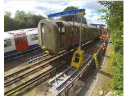
Removal of decommissioned London Tube trains with a hydraulic gantry
