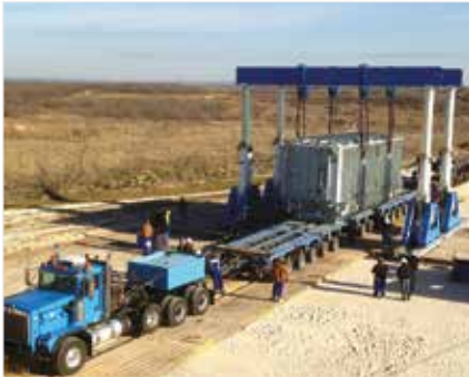
Transformer installation with a hydraulic gantry.
