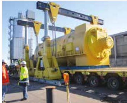
Turbine lift and load-in at a shipping port.
