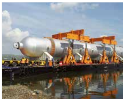
Using two SBL1100 gantries for offloading a 1300 ton hydrocracker
