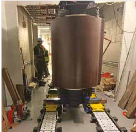
The Enerpac Low-Height Skidding System allows the maintenance team to transport transformers with access limitations.
