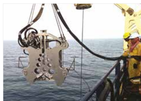
▲ MDWS Diamond Wire Saw lowered into sea.
