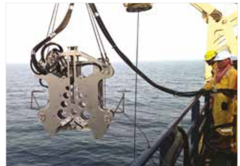
▲ MDWS Diamond Wire Saw lowered into sea.
