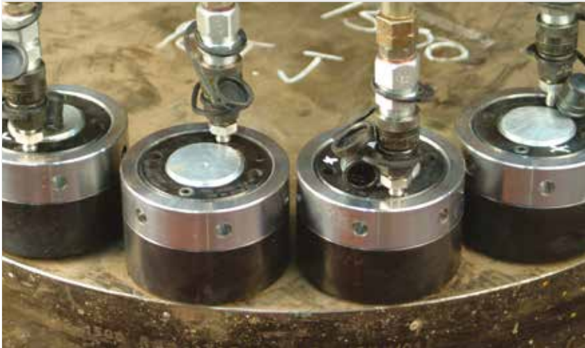
▲ Tensioning with hydraulic nuts.
