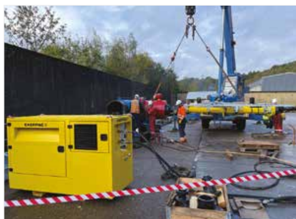
◀ Enerpac MHT2460-H hot tapping machine powered by a PP44-Series Power Pack.
